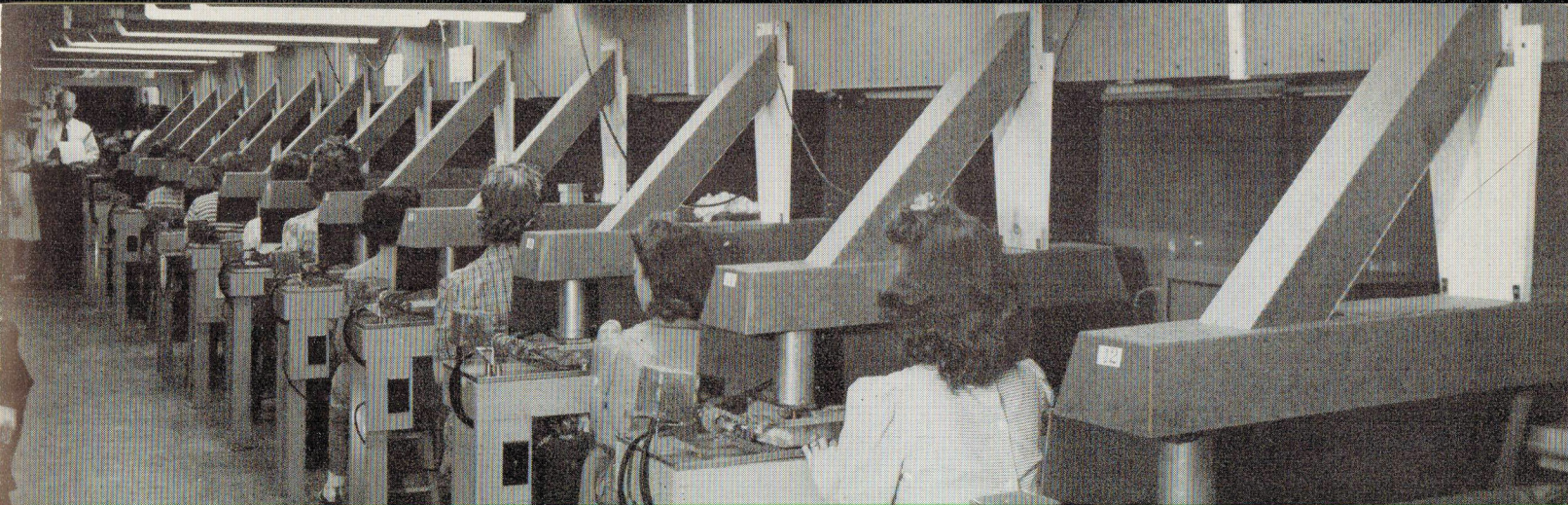
ETCHING PROCESS. HERE CRYSTAL BLANKS ARE BROUGHT TO PREDETERMINED FREQUENCIES BY USE OF ETCHING MACHINES.
