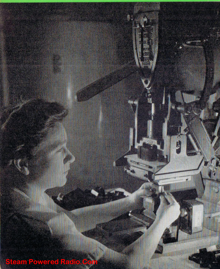
Holder assembly. The pictures appearing on this page were furnished through courtesy of Cryco, Inc., showing assembly of contact plates in plastic holder above, and stamping machine below, engraving identifying marks on the plastic crystal holders.
