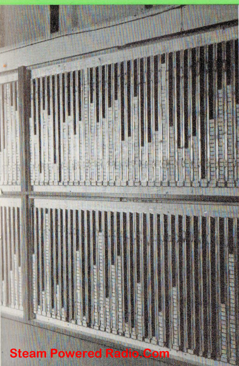
CRYSTAL BLANKS ARE NOW "CHANNELED" OR SORTED AS TO THEIR FREQUENCIES AND ARE GROUPED IN FREQUENCY RANGES OF 25 KC PREPARATORY TO ETCHING.
