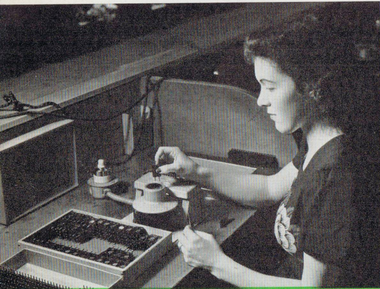
Holder assembly. The pictures appearing on this page were furnished through courtesy of Cryco, Inc., showing assembly of contact plates in plastic holder above, and stamping machine below, engraving identifying marks on the plastic crystal holders.
