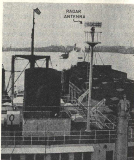
Typical radar antenna installation.
